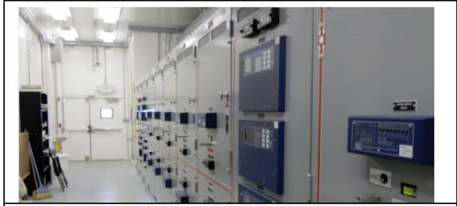
**New switchgear installed at the central power plant. This switchgear allows the CHP project to meet critical loads when switching to island mode operation.**
