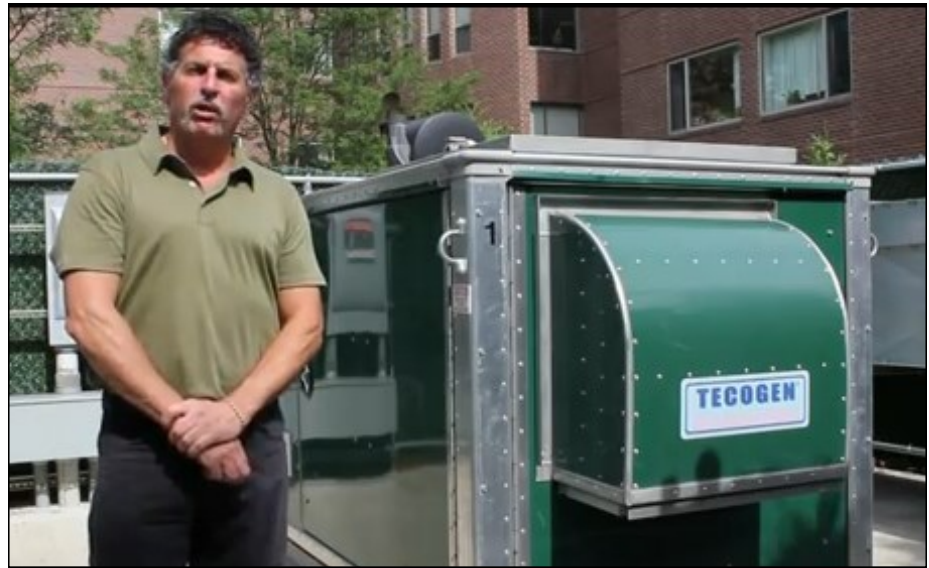
Gregg Giampaolo explains the benefits of the Gurwin project. His company, All Systems Cogeneration, did the engineering for the project.
