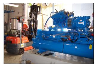
The placement of the Tecochill Natural Gas Engine Driven Chiller is now complete and all that is needed is to install the sound attenuating engine enclosure and make the final connections.
