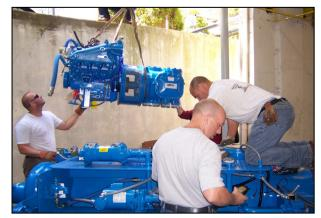
**3.** Once inside, the engine/compressor assembly is reassembled above the condenser and evaporator.
