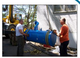
2. The refrigerant oil separator is rigged into the basement mechanical room to be assembled onto the chiller.
