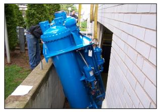
1. The evaporator and condenser assembly are rigged through the ventilation louver that was originally used for combustion air for the boilers.
