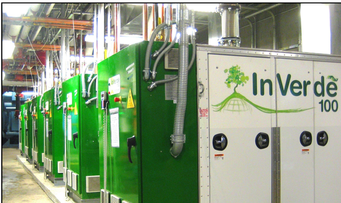
Six Tecogen INV-100s, create 600kW of power on-site to keep Manhattan Beer Distributors operating efficiently and cost effectively.
