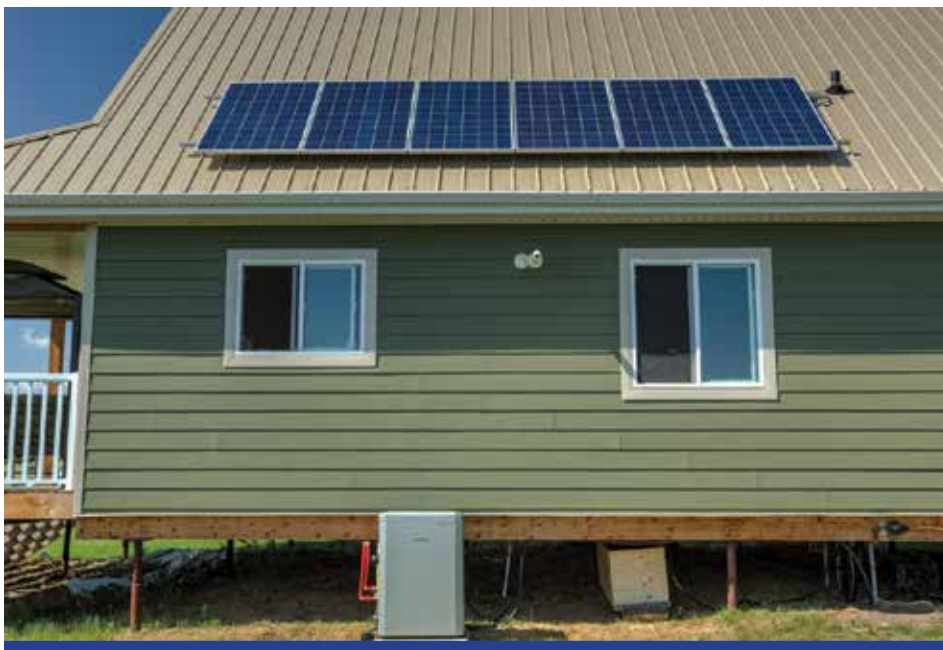
This house in Edmonton, Canada, twinned solar photo-voltaic roof panels with microCHP (combined heat and power) to increase efficiency, slash fuel consumption and lower greenhouse gas emissions by 55 percent.
