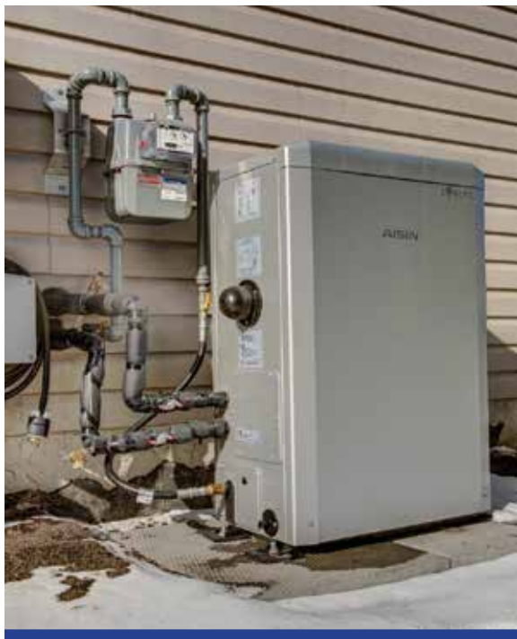
The home in Edmonton, Canada, is powered by an Aisin 1.5 kilowatt natural gas engine. The waste heat is used to heat water as well as for space heating.
