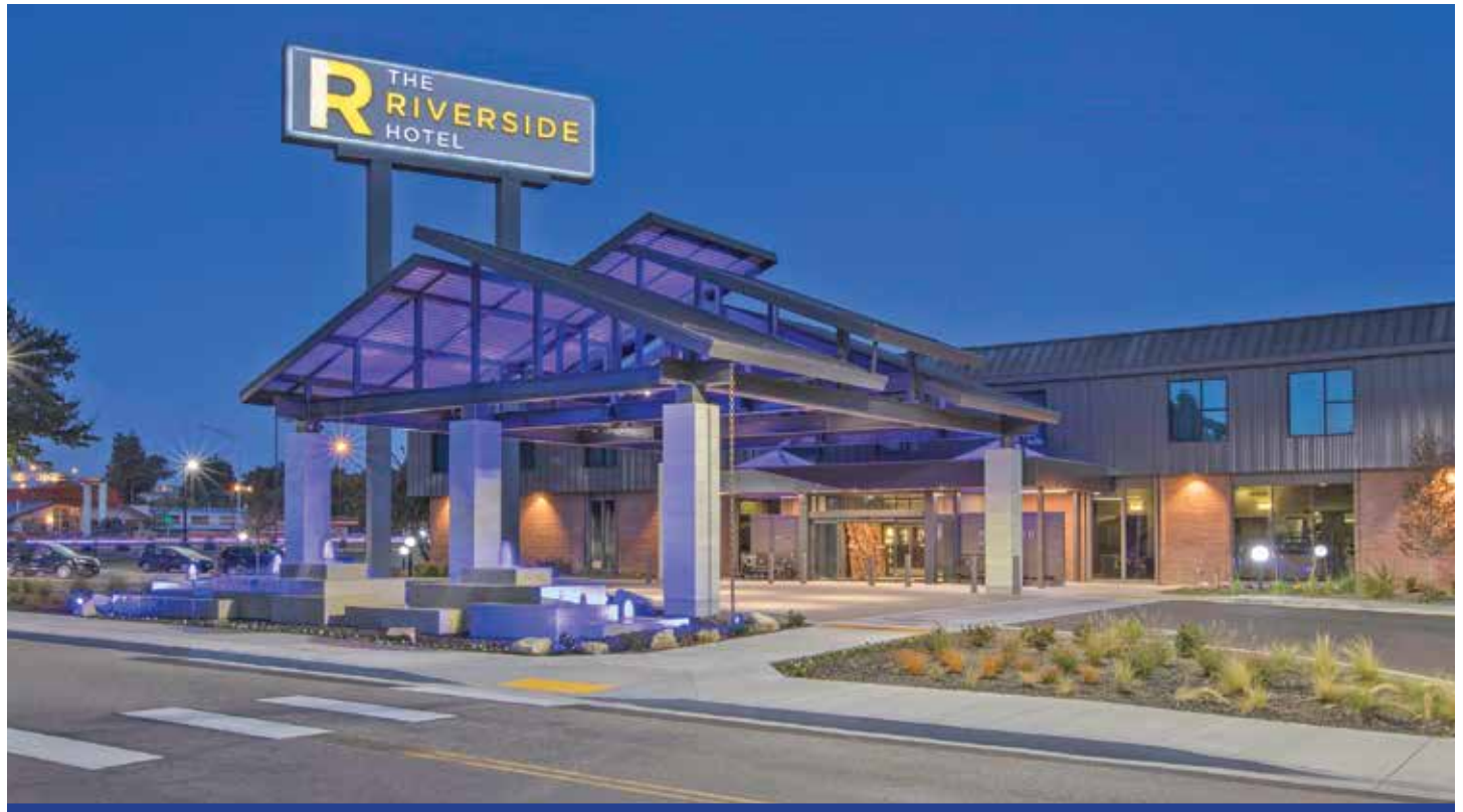
The Riverside Hotel — the largest in the Boise, Idaho, market — installed a new combined heat and power (CHP) system offering cost-effective and energy-efficient generation of electricity, heat and hot water as part of its renovation of the 300-room property.
