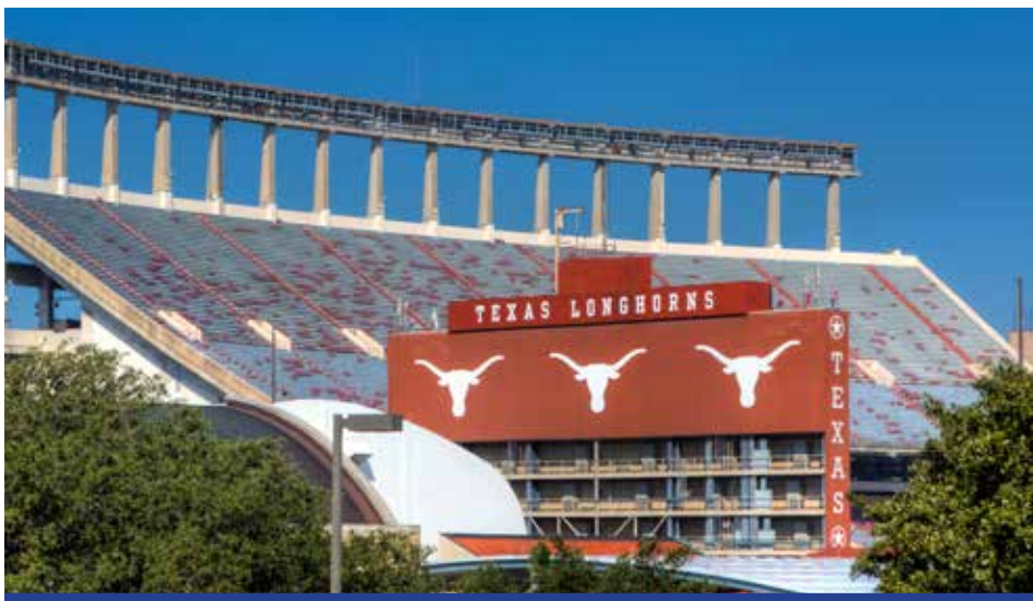
The University of Texas Austin (above) has a CHP plant that provides all campus electricity, heating and cooling for more than 150 campus buildings serving 70,000 faculty, students and staff.
