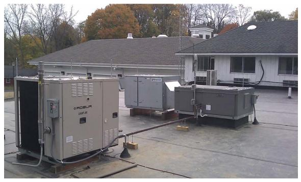
The Robur gas heat pump above is piped to an air handler that is connected to an energy recovery ventilation unit (ERV). Return air from the space is used to warm and cool the ventilation air, thus reducing energy costs to heat and cool the incoming outside air.
