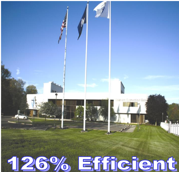
Southern Connecticut Gas installed 5 GAS HEAT PUMPS In their own facility in Orange, CT .
