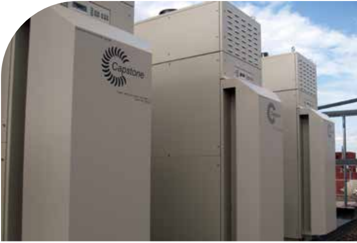
Commissioned in 2019, the rooftop-mounted C65 ICHP microturbines have logged more than 85,000 runtime hours, which amount to 99.8% uptime.
