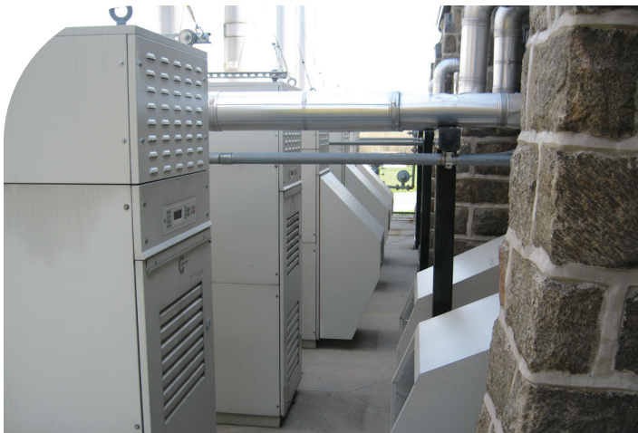
Capstone microturbines generate electricity and heating at Masonic Village, a 1,400-acre complex serving more than 2,000 residents since 1910.
