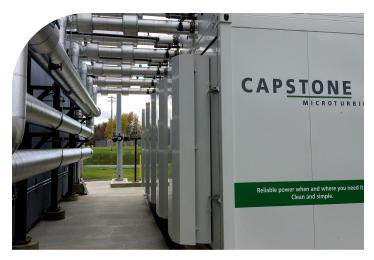
A Capstone C1000S microturbine in a combined heat and power (CHP) application supply the industrial R&D facility's electrical and hot water heating needs.
