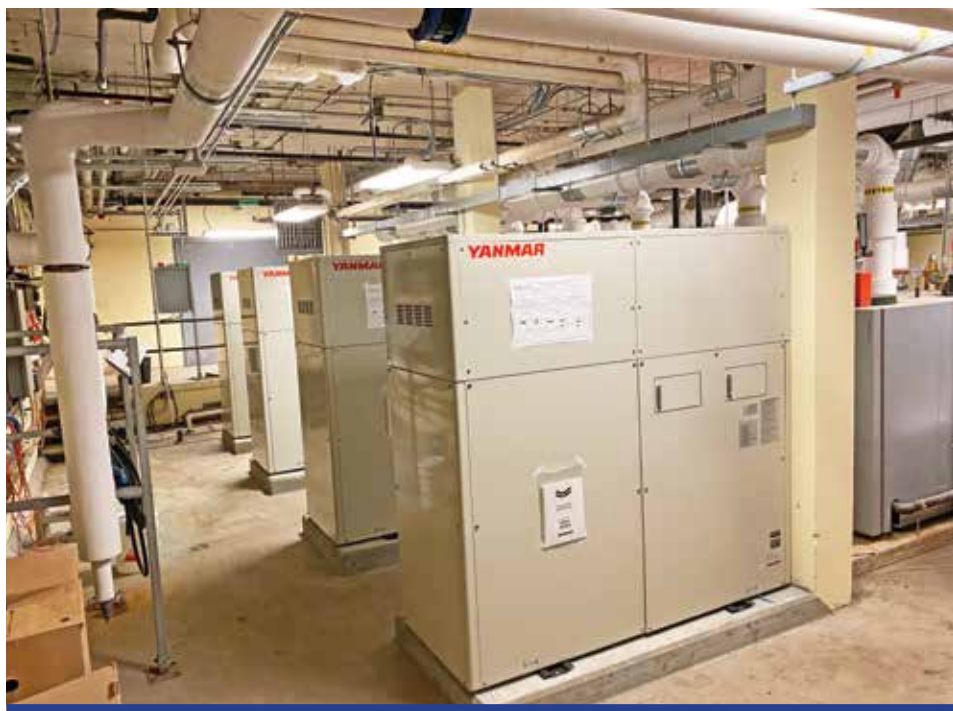
At Naugatuck High School, a cogeneration installation will provide 140 kilowatts of electrical power and 820,000 British thermal units of hot water to supply heat.
