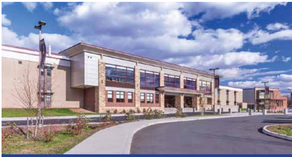
At Naugatuck High School in Naugatuck, Connecticut, a cogeneration installation will provide 140 kW of electrical power and 820,000 British thermal units of hot water to supply heat for the school's domestic needs and an Olympic-size indoor pool.
