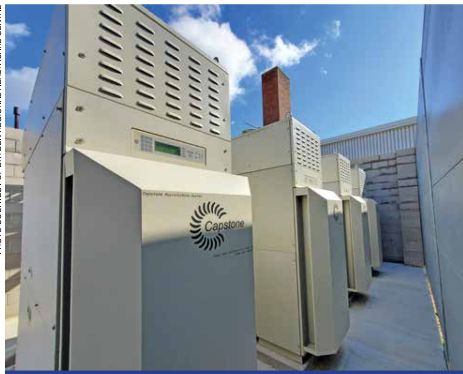
Dryden Regional Healthcare Centre turned to CHP to reduce its rapidly increasing electricity costs. Four natural gas-fueled Capstone C65 microturbines provide electricity and supply the building’s heat, leading to cost savings of at least $150,000 per year.
