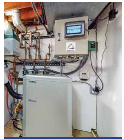
Aisin World Corp. of America provided a micro combined heat and power unit to a residential unit in Michigan capable of generating up to 1.5 kilowatts of power.
