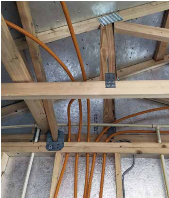
Corrugated stainless steel tubing, or CSST, has replaced iron and copper pipes as a way of delivering natural gas and propane to residential and commercial facilities due to its greater safety and ease of installation.
